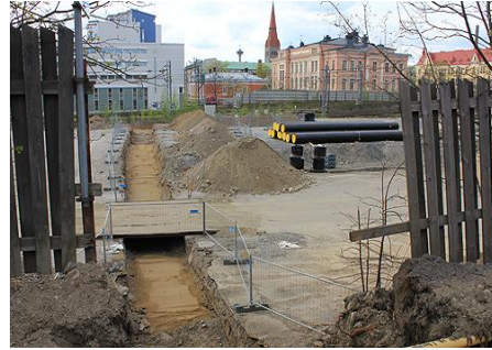
Building of the district cooling network, started in 2012 (8.5 km so far)
