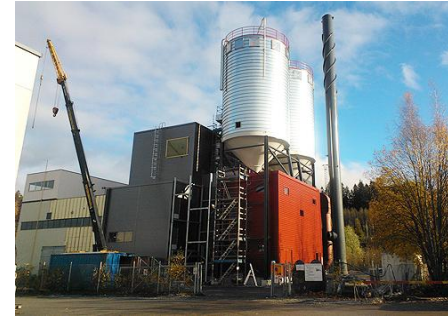
Largest pellet heat plant in Finland, 10 MEUR
